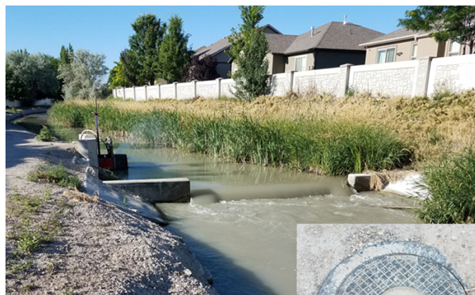
A Typical Urban Secondary Water Diversion with a Flow Meter Only at the Diversion, Salt Lake County, Utah
